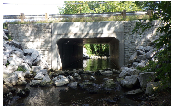
Harrison Road over Dry Run after construction 2023
