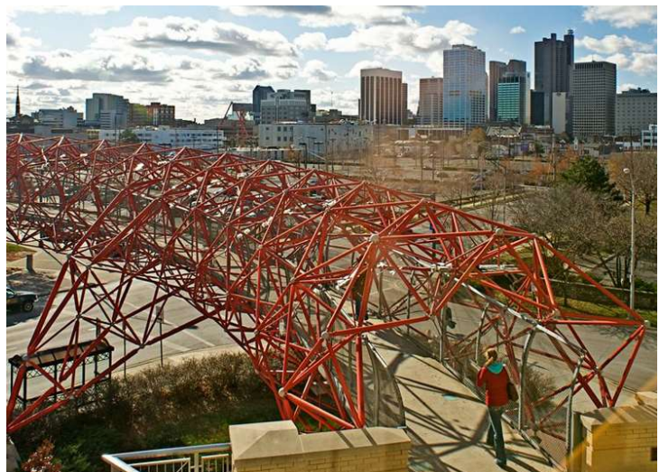
Columbus State Community College pedestrian bridge over Spring Street
