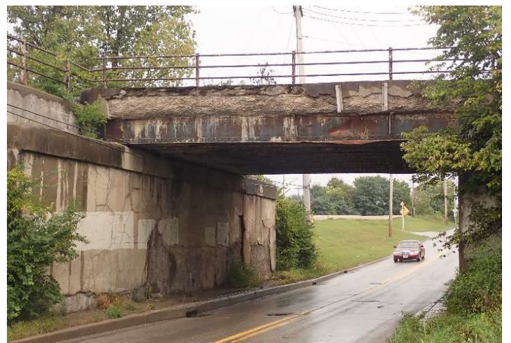
Bridge over Williams Rd under CSX
