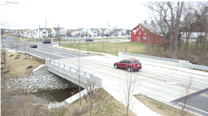
Lehman Rd. over Pickering Creek
