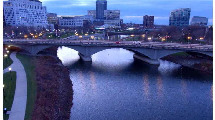
ODOT Bridge on US-40 Broad Street over Scioto River
