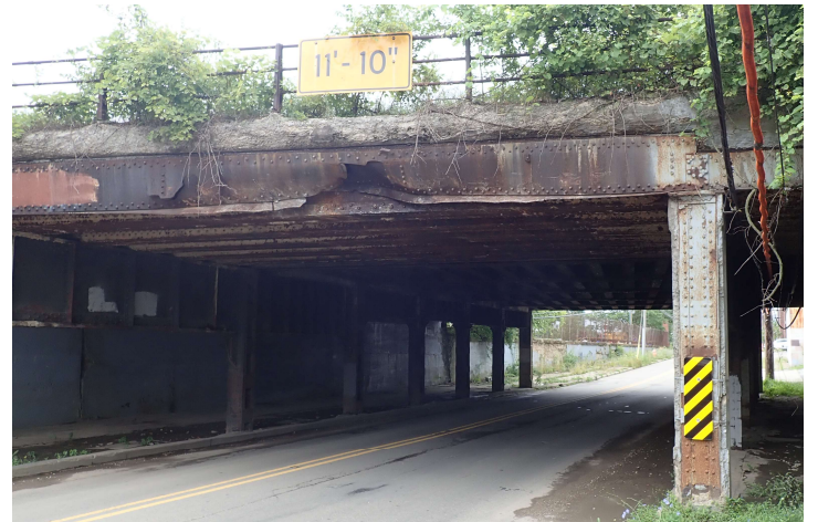
Bridge over Second Ave under CSX
