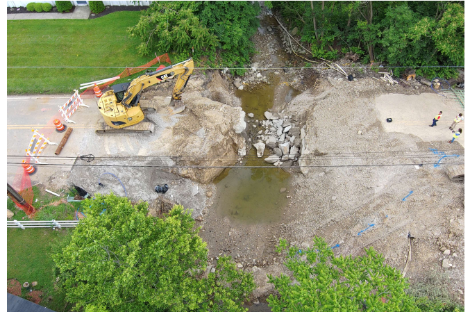
Harrison Road over Dry Run during construction 2022
