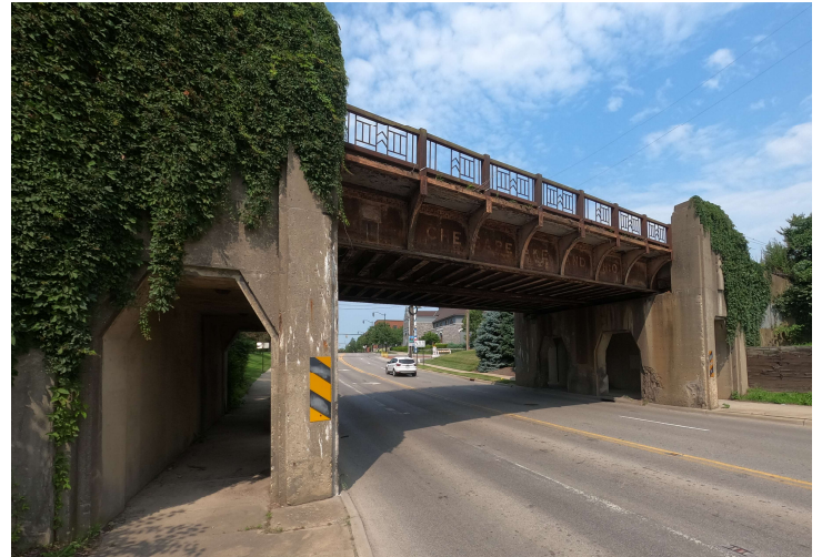
Bridge over Goodale Ave under Norfolk Southern
