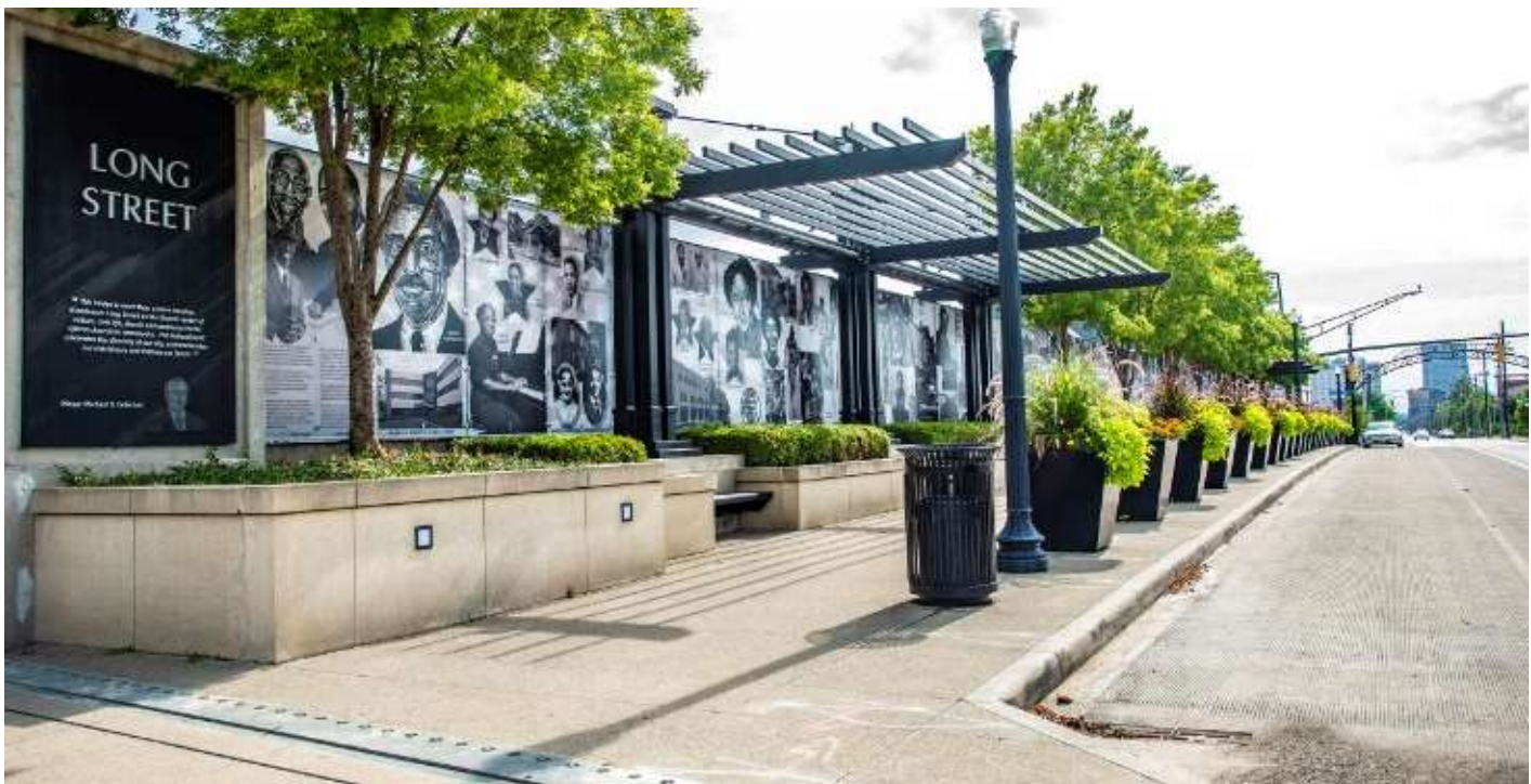
Bridge on Long Street over I-71, ODOT owns the roadway bridge, City owns the park cap bridge.
