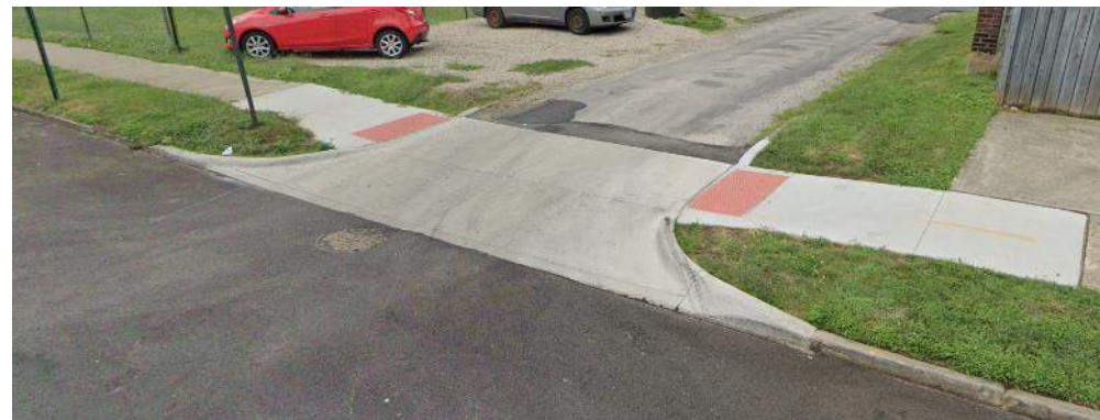
Blended transition at a raised PAR
