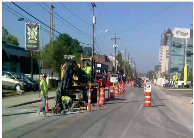
Roadwork along Livingston Ave.
