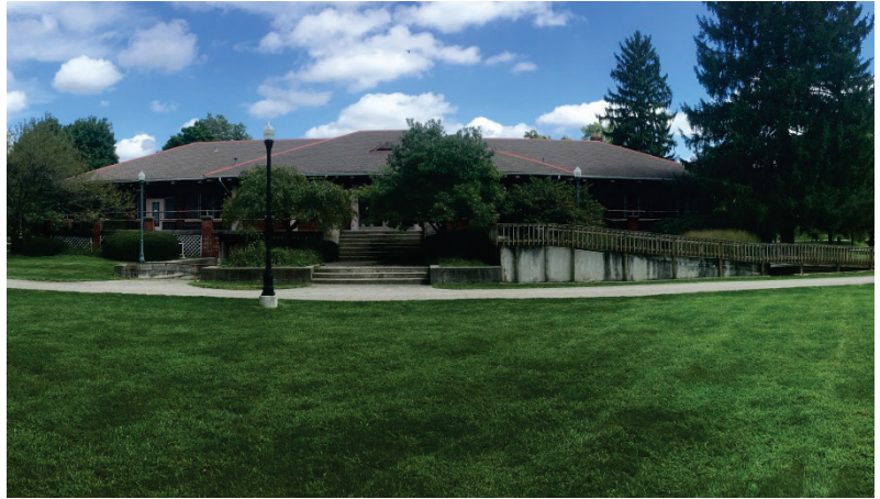
Existing exterior of the Davis Center.
