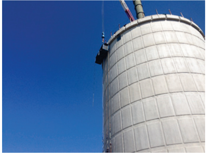
Completed concrete column of new composite elevated storage tank.
