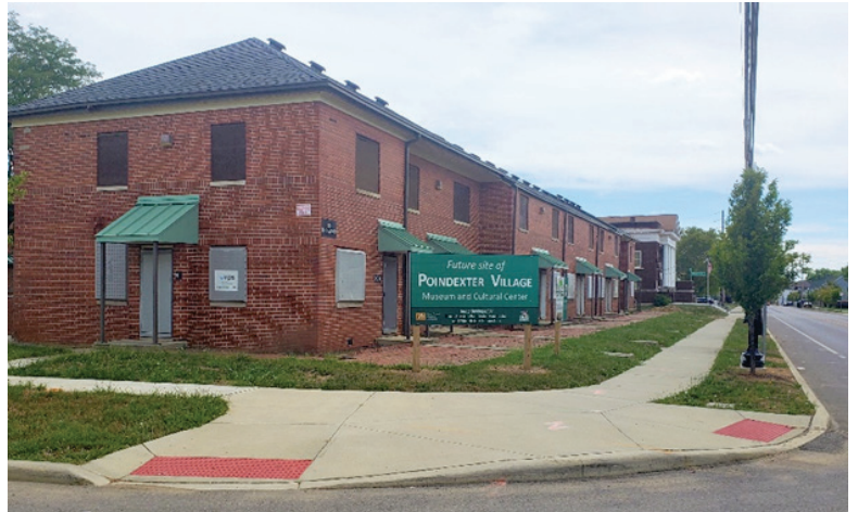
Project is currently under construction/redevelopment.
