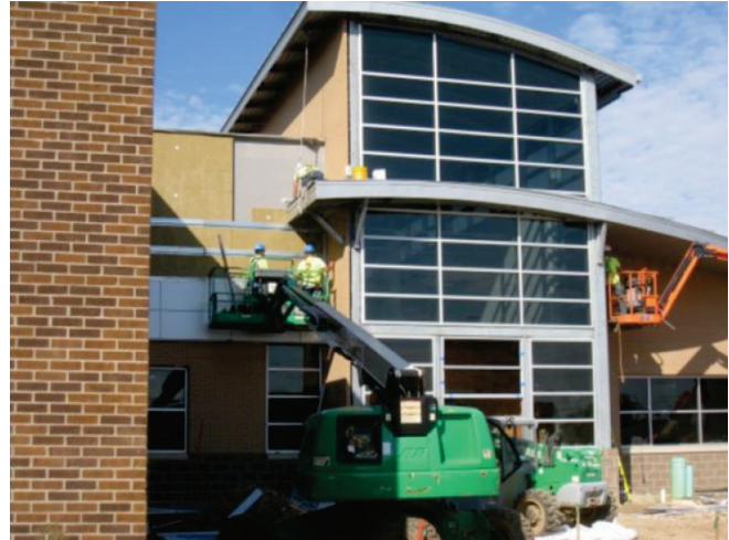
Photograph of the construction at Indian Mound Recreation Center.
