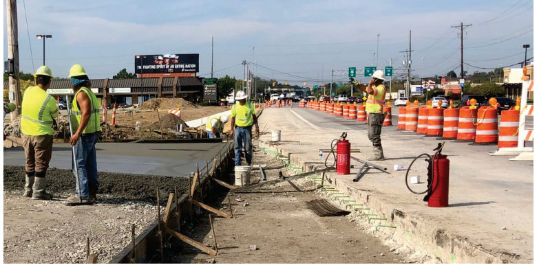
Construction In progress.
