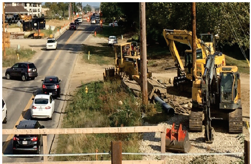
Construction in progress on Lazelle Road.
