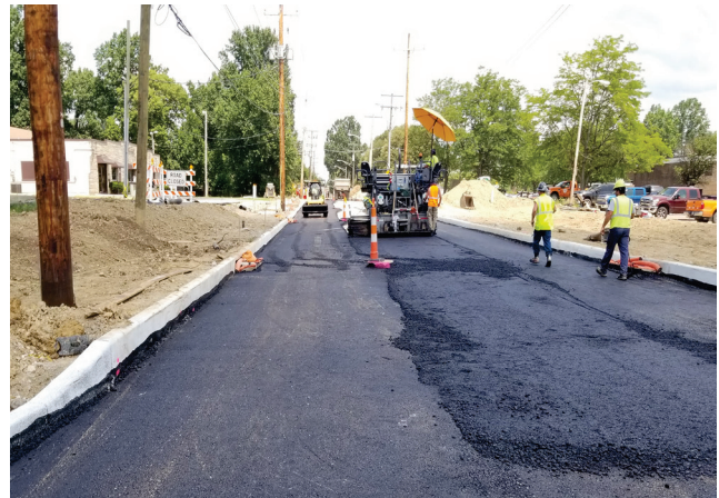
Roadway work at Barnett and Livingston.
