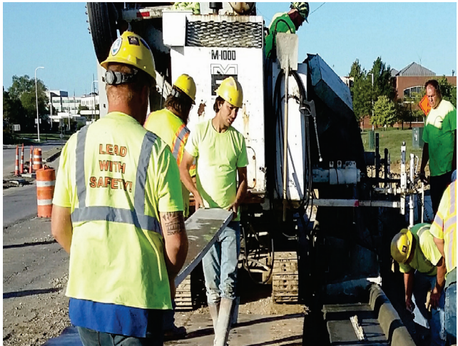
Curb Installation on Polaris Parkway
