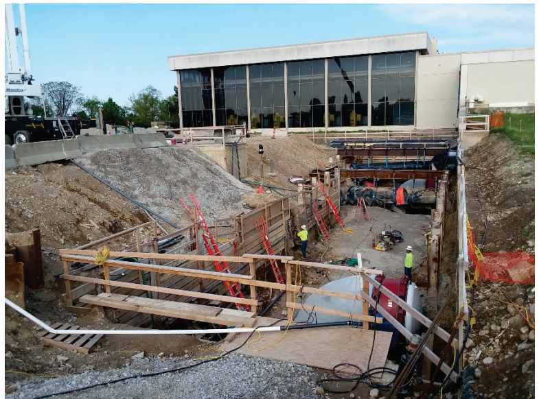
Excavation for the new DRWP UV Disinfection Facility
