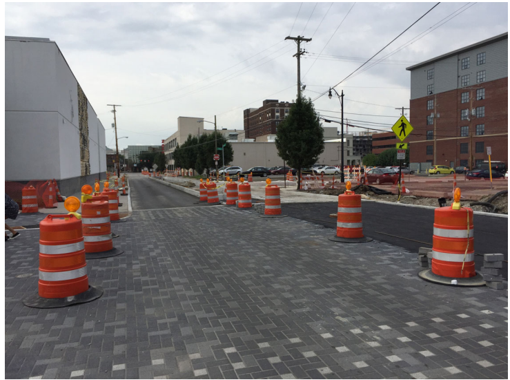
Roadwork along Cleveland Ave.
