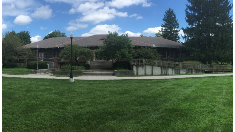
Davis Center existing exterior.
