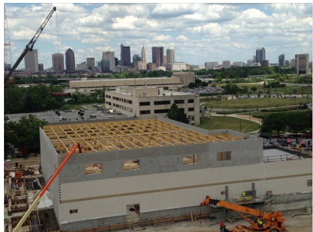
Construction of the new ion exchange facility.
