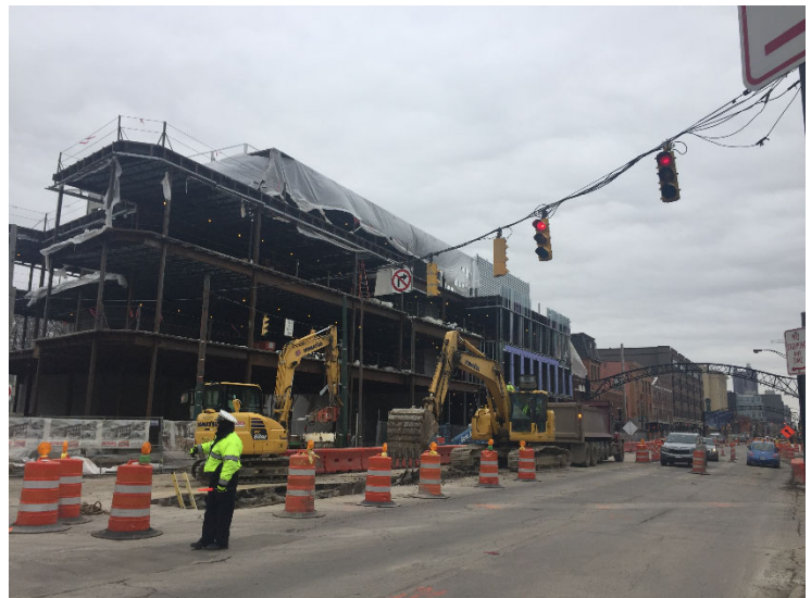
Roadway work along N. High Street.
