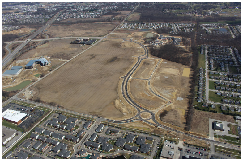
Aerial photograph of the completed construction of the N. Hamilton Road “S” curve at State Route 161.
