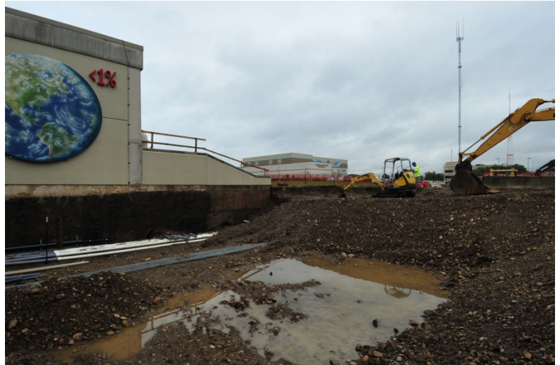
Excavation begins for the new DRWP UV Disinfection Facility
