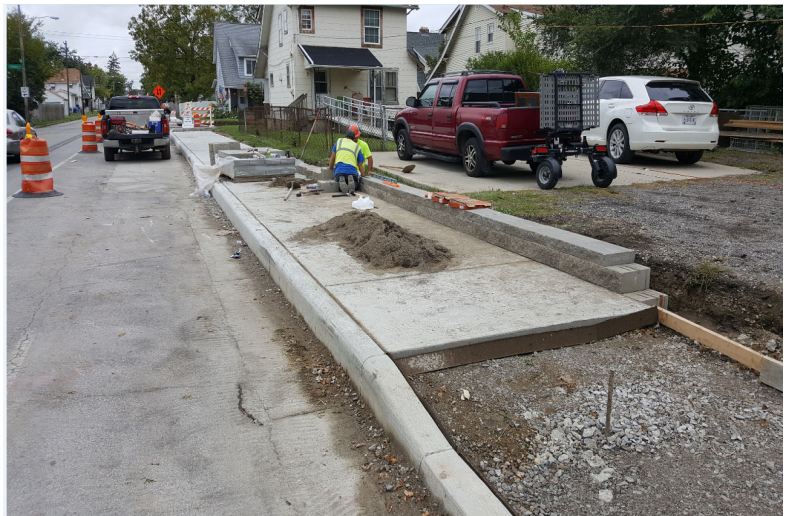
Installing sidewalk on W. Mound Street near S. Terrace Ave.
