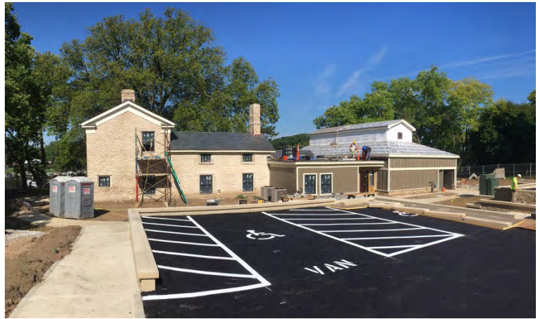
Lashutka Event Center, currently under construction. Projected completion date of November 2016.
