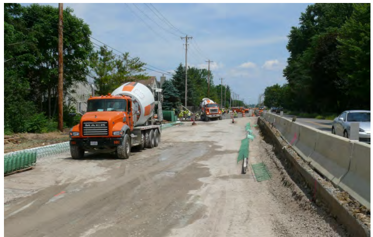
Photograph of roadwork preparation for the Hard Road project.
