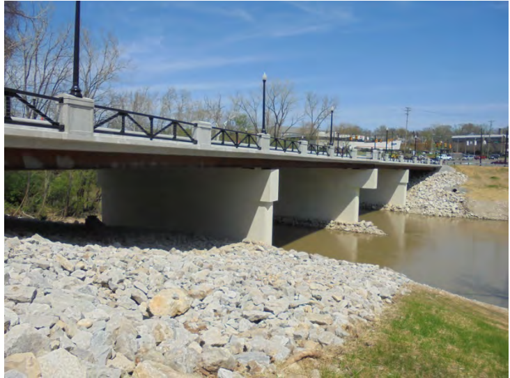
The newly constructed Fifth Avenue bridge over the Scioto River.
