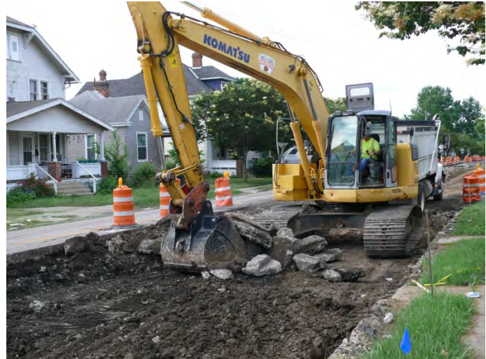
Removal of existing roadway to prepare for improvements along Hague Avenue.
