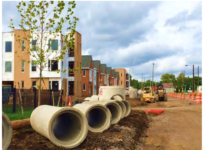
Photograph of the newly added housing units in the Poindexter Village area, currently under construction.
