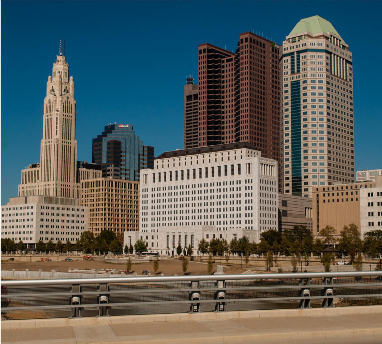
Present day view of Rich Street Bridge. The city closed the Town Street bridge in 2008, realigned it, and reopened it in 2011 as Rich Street Bridge. The bridge is 568 feet in length, 37 feet in width, and has 10-foot wide sidewalks on both sides.
