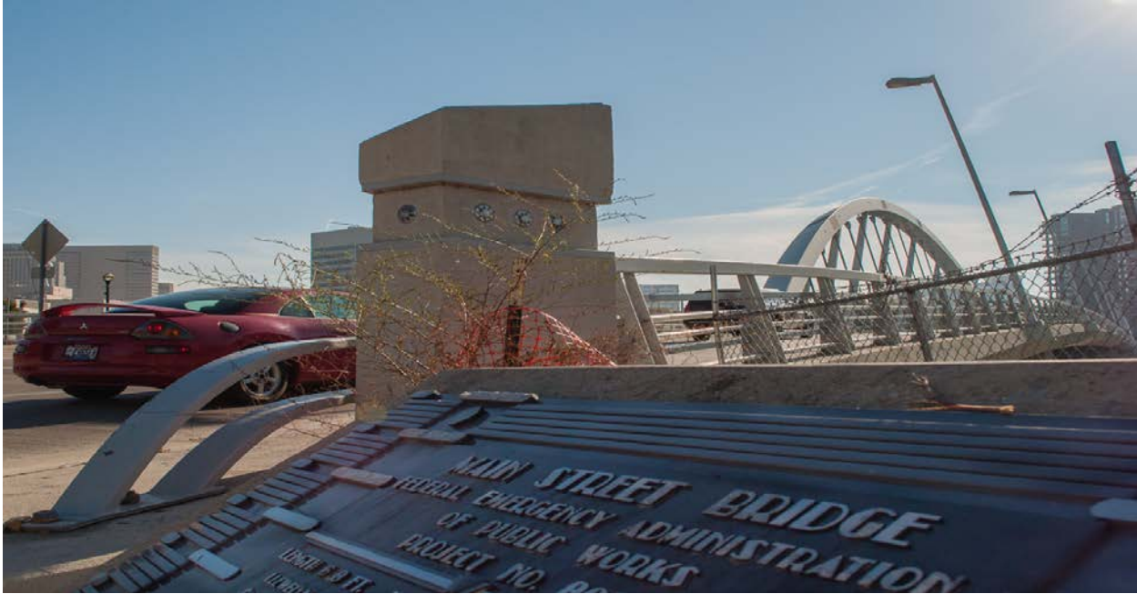
Present-day view of Main Street Bridge. The bridge's arch in the background at its peak is 65.5 feet above the road deck.
