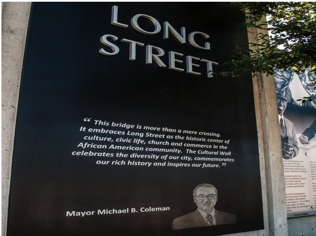
The Long Street Bridge cap includes a landscaped pedestrian walkway and features images, past and present, honoring people, places and institutions that have made an impact on the King-Lincoln and Discovery Districts.
