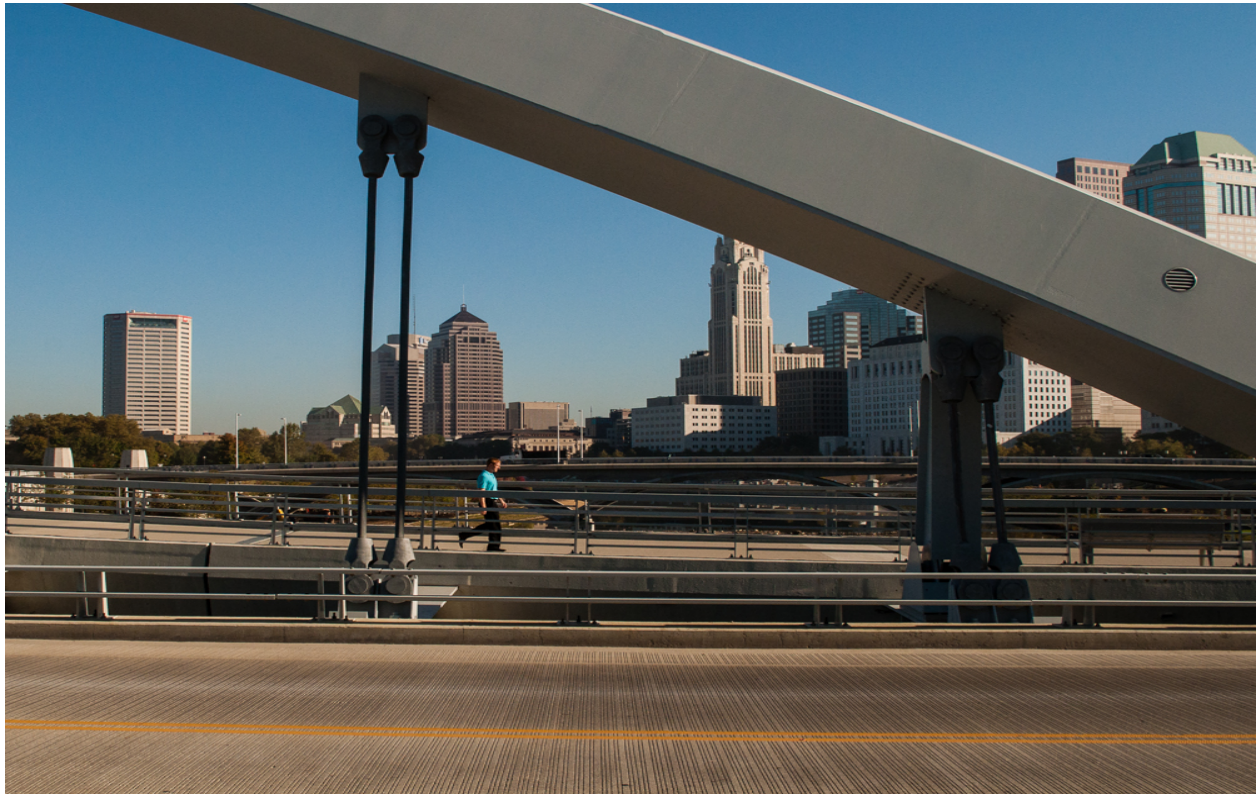
View of the present-day Main Street Bridge looking north into downtown. The bridge connects the Franklinton neighborhood with Downtown and includes an 18-foot, 7-inch wide multi-use path to accommodate pedestrians and cyclists.
