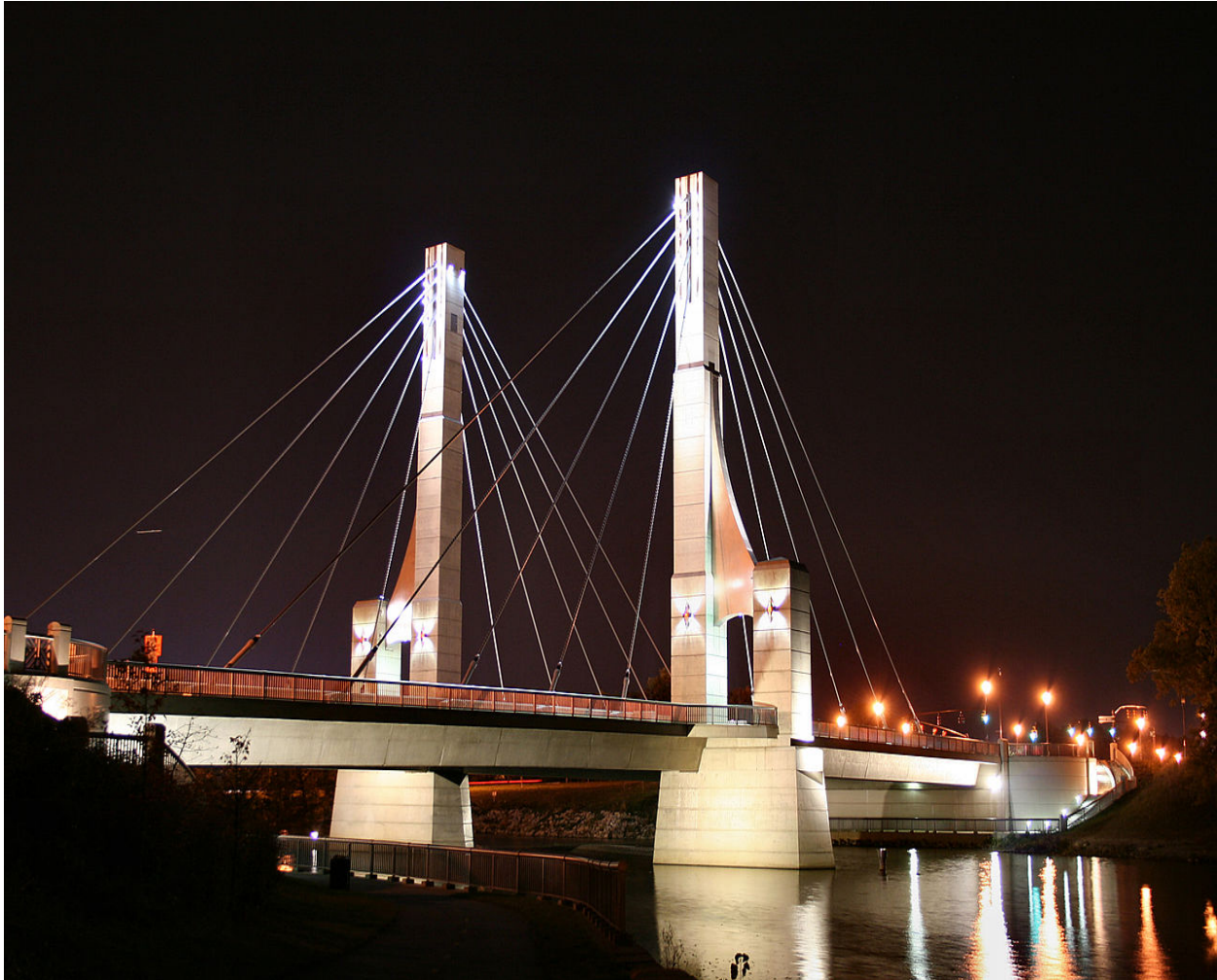
A night view of the Lane Avenue Bridge spanning the Olentangy River. The bridge was completed in November of 2013, five months ahead of schedule. The Lane Avenue Bridge was built as a replacement for its predecessor, a concrete earthen bridge that had originally opened in 1919.
