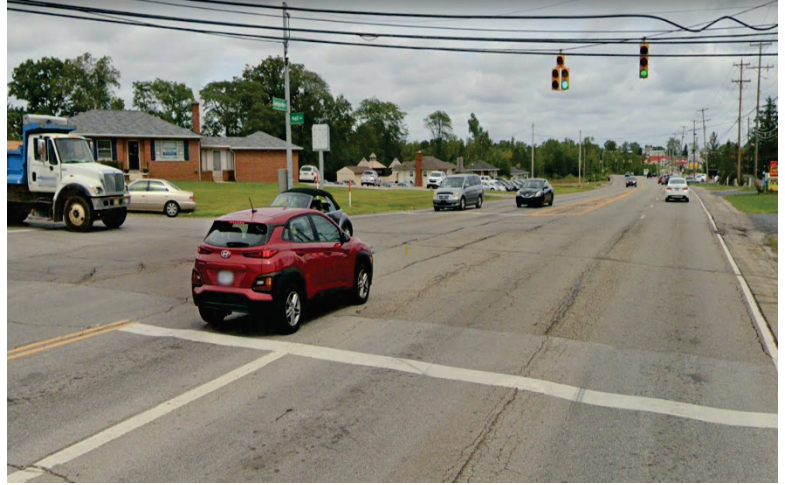
View of Georgesville Road at the intersection with Hall Road
