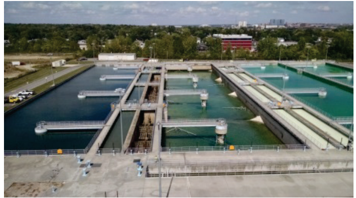
Existing treatment basins and clarifier equipment will be replaced under this project
