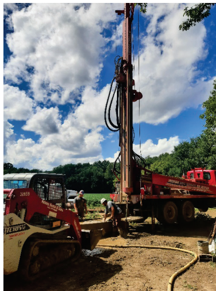
View of the PAWP Collector Well 112 test well being drilled
