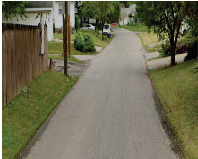
Section of Grace Street to receive sidewalks
