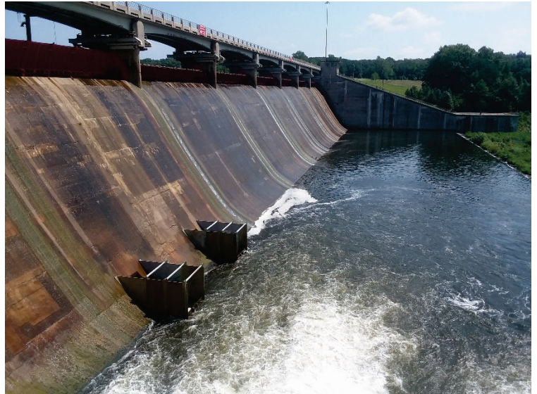
View of Hoover Dam spillway showing the temporary cascade aerators installed under this project
