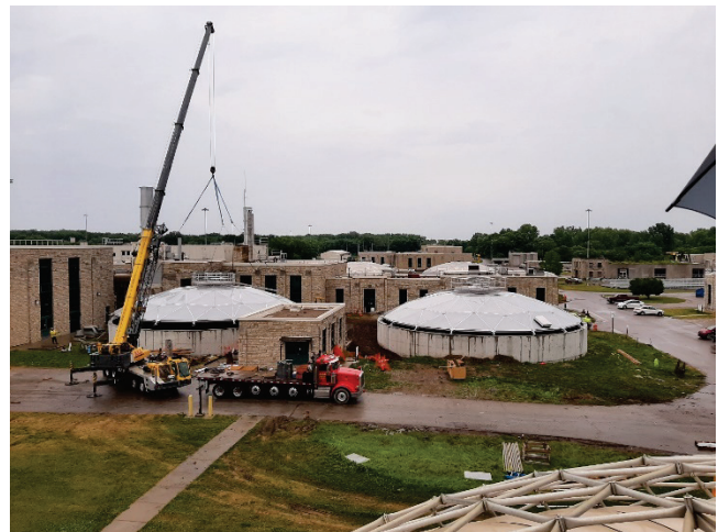
View of the Jackson Pike Wastewater Treatment Plant.
