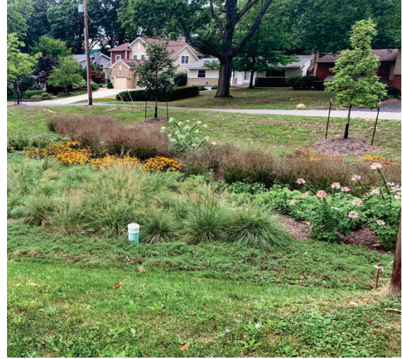
Completed regional bioretention basin.
