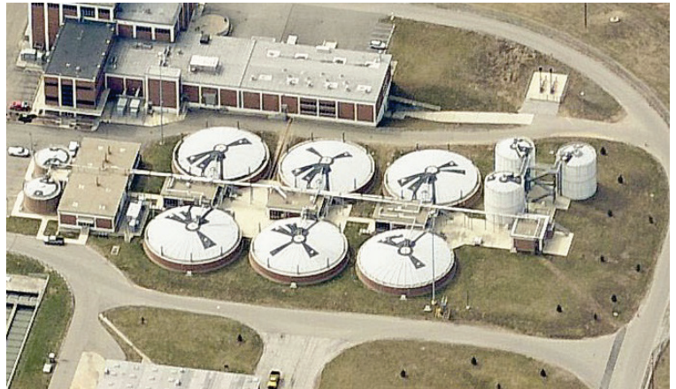
View of the current digesters at the Southerly Wastewater Treatment Plant.
