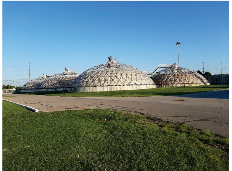
Digesters at the Jackson Pike Wastewater Treatment Plant
