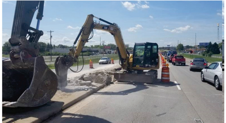
Removal of median on Hamilton Road just north of Groves Road
