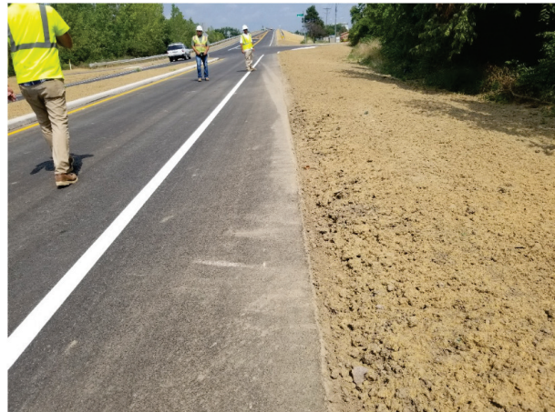
Finishing construction of the Wilson Road Shared Use Path
