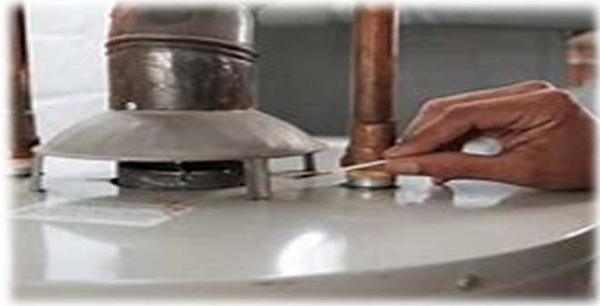
A properly vented hot water tank should draw the smoke from a match up and out of the vent as shown in the picture.
