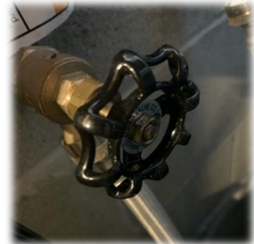
Turn these handle valves clockwise to close, and counterclockwise to open
