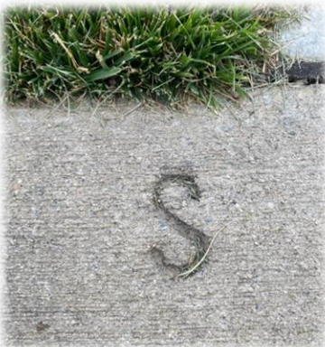
The "S" stamped in the curb shows the general location of the sewer line
