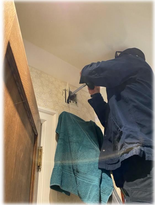
This shows a firefighter using the manual override rod (see photo on previous page) to lower the car
