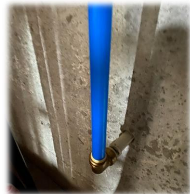
Locating the main water into the home and the W on the curb can help to locate the water box
