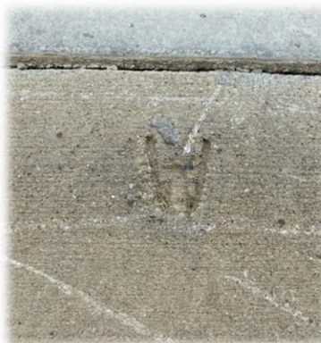
The "W" stamped in the curb shows the general location of the water line
