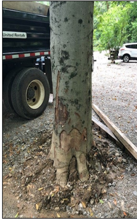
Figure 4: Beech tree in Beechwold Nature Preserve with trunk damage from nearby construction. Truck parked in CRZ is also compacting soil and roots.
