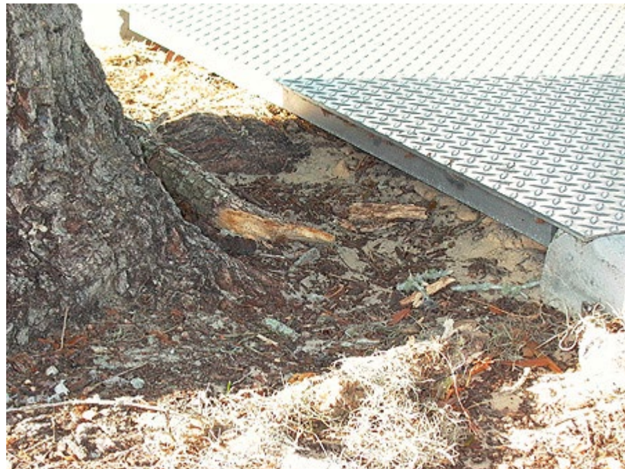
Figure G7. Sidewalk bridging over tree roots. Photo: Edward F. Gilman, Professor, Environmental Horticulture Department, IFAS, University of Florida
