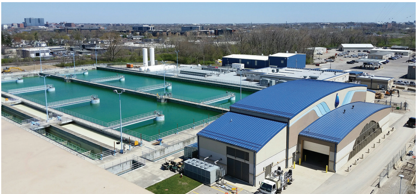
Dublin Road Water Treatment Plant
