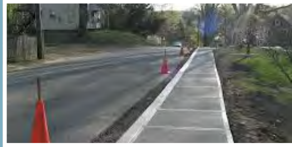
INSTALL MISSING SIDEWALKS
