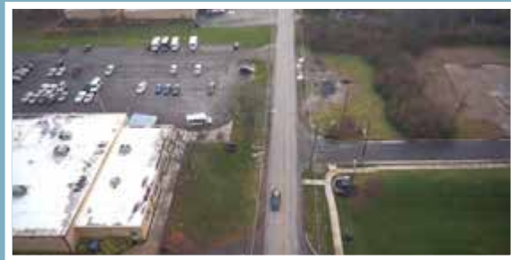
HARMON AVENUE CORRIDOR
