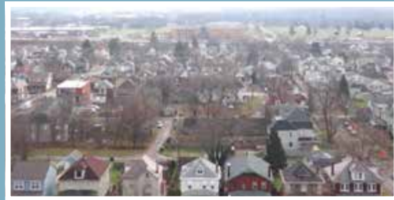
MISSING SIDEWALKS SOUTH OF SULLIVANT
