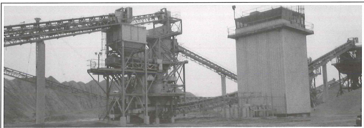
Sand and gravel aggregate processing at the Olen Corporation.
