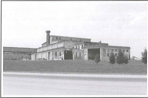
Hartman Dairy Complex, built in 1903, was the largest dairy operation of its kind.
