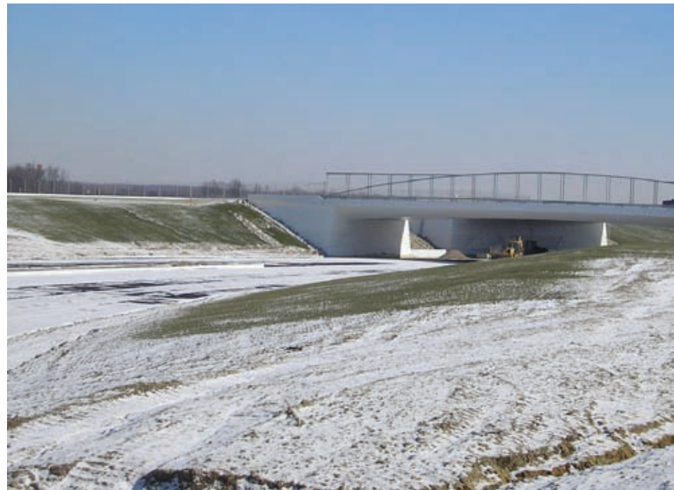
The new Crossover Taxiway under construction.
