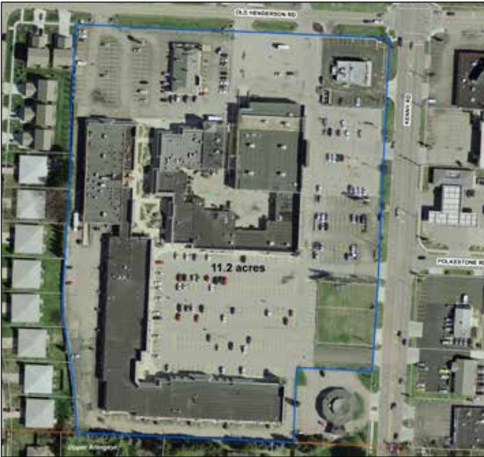
Top: View of Kenny Centre from across the street. (Source: Google Maps) Bottom: Aerial view of Kenny Centre
