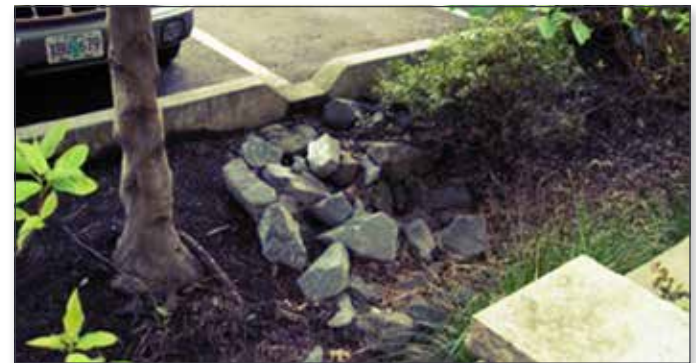
Bioswale used to capture rainwater from a parking lot.
