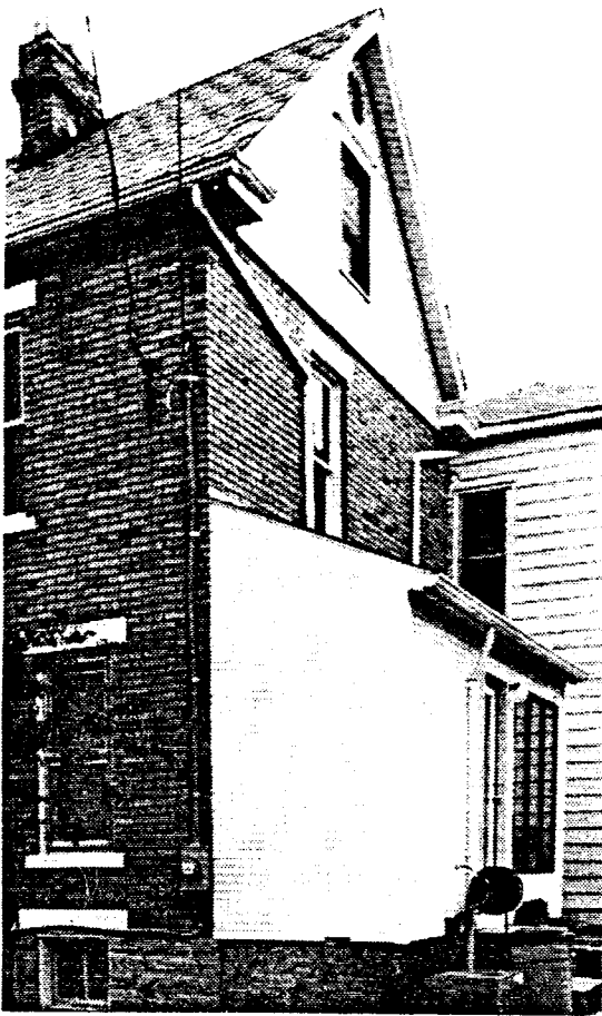
68 E. Lincoln Street Frame Addition
