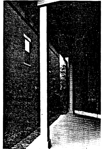
108 E. Lincoln Street Replacement columns
