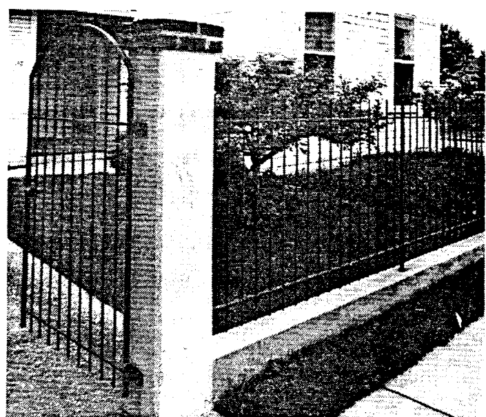
24 E. Lincoln Street (New Fence)
