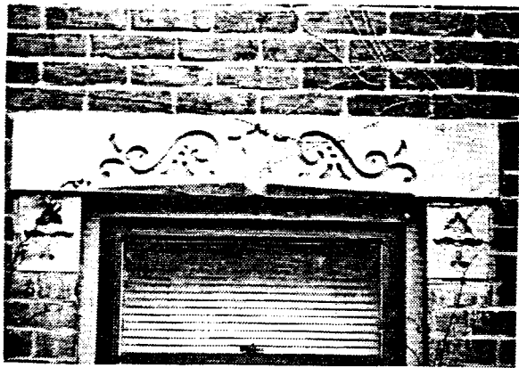
97 E. Lincoln Carved Lintel & Hoodmolds
