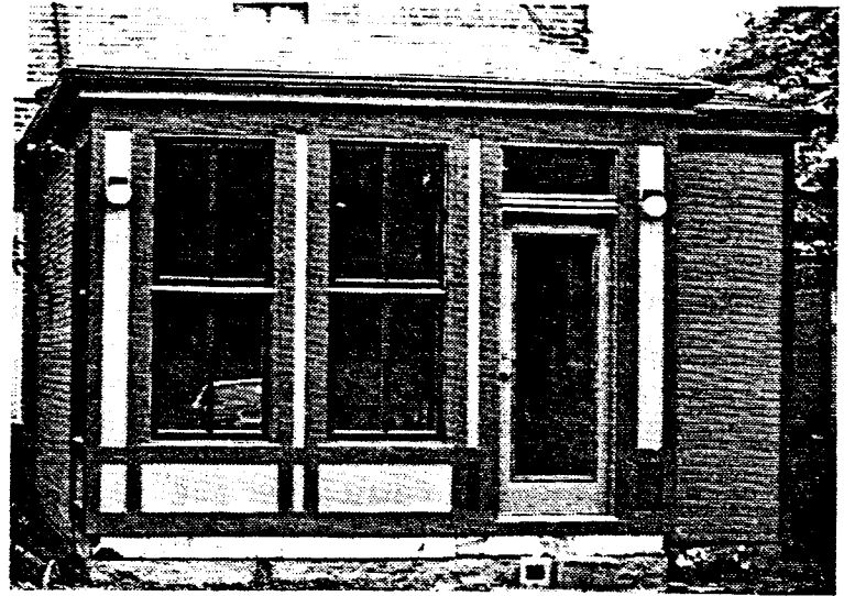
84 E. Lincoln Street Frame Addition
