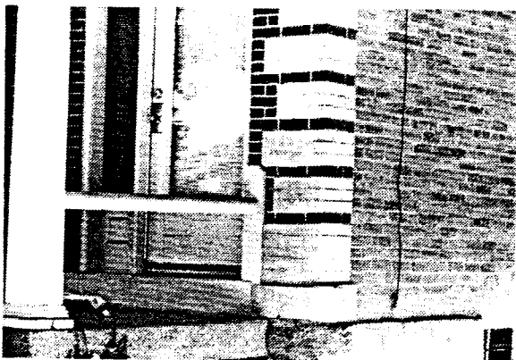
31 E. Second Avenue Light & Dark brick on front of building, with common brick used on sides & rear
