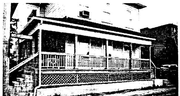
40-41 E. Second Avenue New Porch
