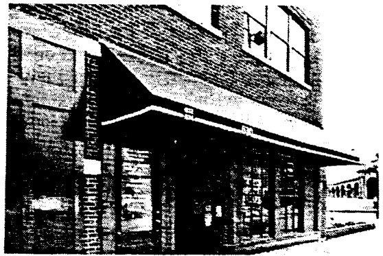
630-634 N. High Street Awning Sign
