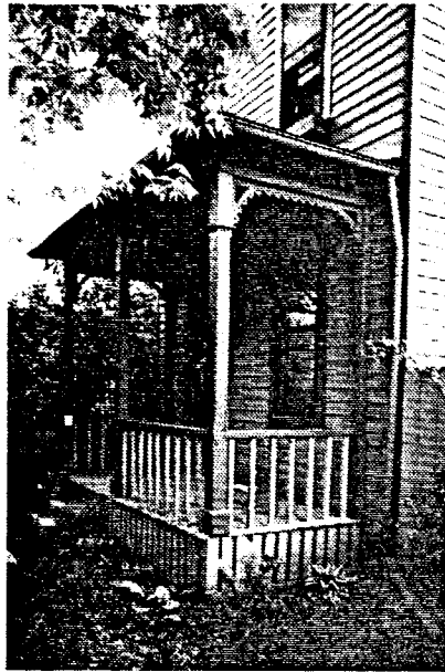
837 Hamlet Street Original porch with replacement balusters, rails and decking
