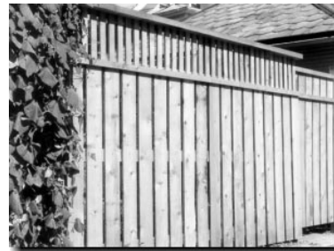
{ PHOTO 70 } This board-on-board six-foot privacy fence has a top fence detail that helps break up the horizontal plane. Also, the “dressed” side of the fence is facing out and the framing is toward the inside.
