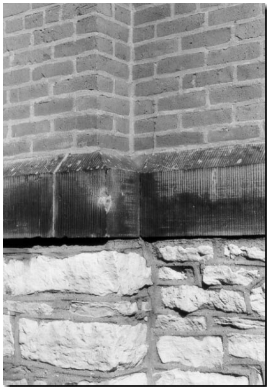
{PHOTO 1} Limestone water table between stone foundation and brick wall.
