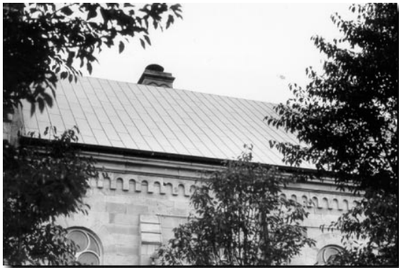
{ PHOTO 23 } Standing seam metal.
