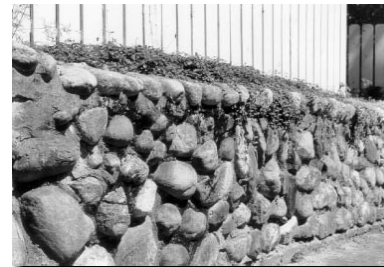
{ PHOTO 82 } Mortared field stone retaining wall.
