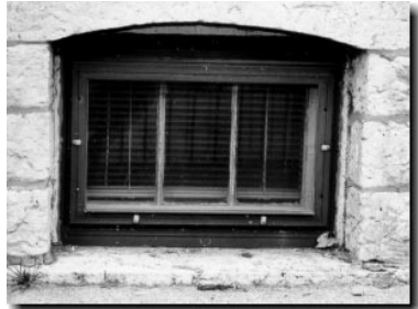
{ PHOTO 39 } Small foundation window with a fixed metal storm.
