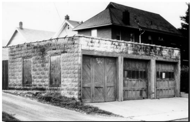
{ PHOTO 84 } Rusticated concrete block garage.
