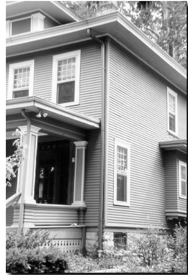
{ PHOTO 29 } Here a downspout is located along a corner board. When possible, locate it along the side or rear of a building.
