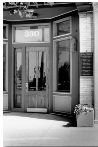
{ PHOTO 62 } Wall mounted sign.
