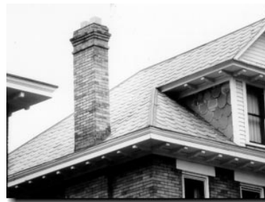
{PHOTO 30} Nicely preserved brick chimney. It has a corbeled top.
