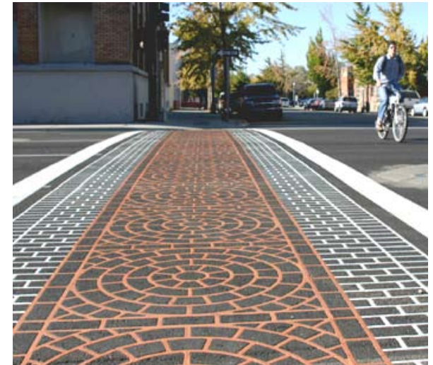
Example of textured cross walk pavement.
