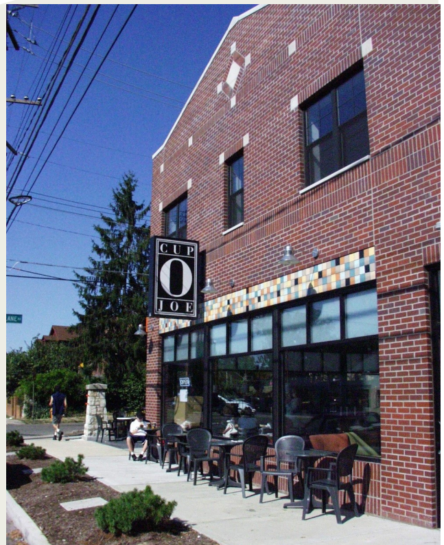
This building illustrates several design guidelines recommended in this plan.
