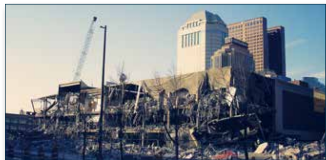
Demolition of the City Center
