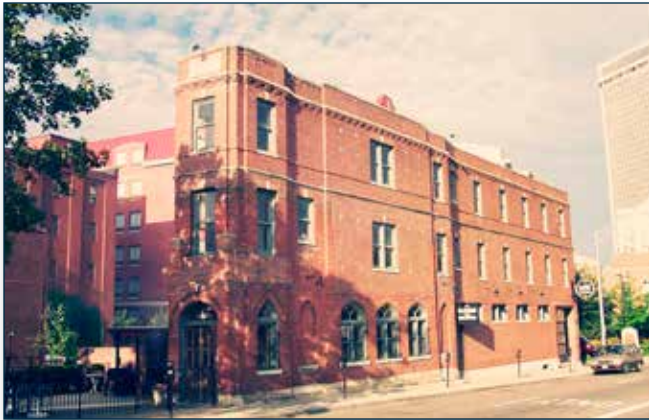
Outdoor dining is provided adjacent to this building as part of the Flatiron Restaurant on Nationwide Boulevard. This is a creative use of available space on the parcel, outside of the right-of-way
