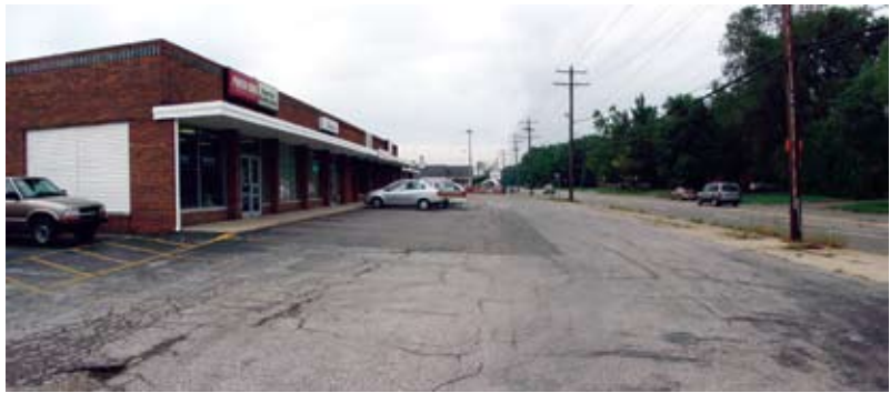
Indianola Avenue at Wetmore Road - Before
