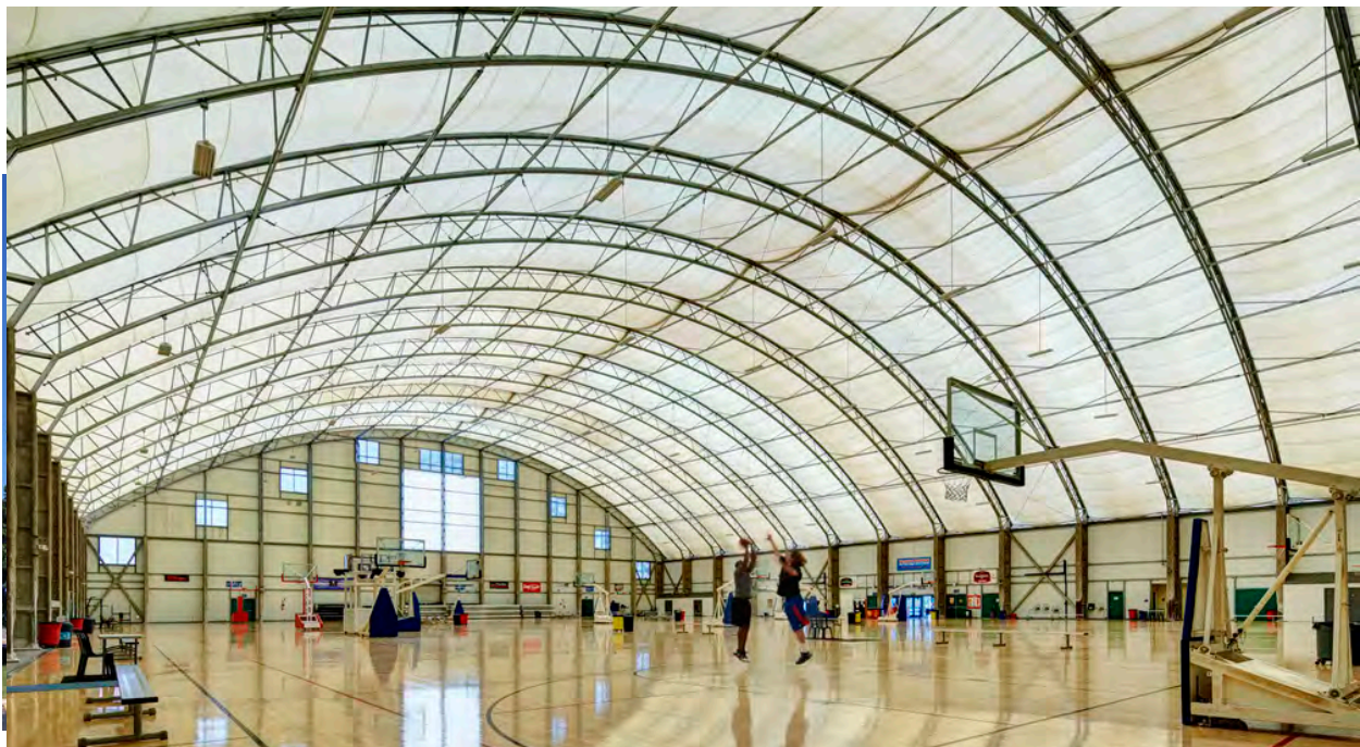
Alliant University Sports Complex; Source: Davy Architecture
