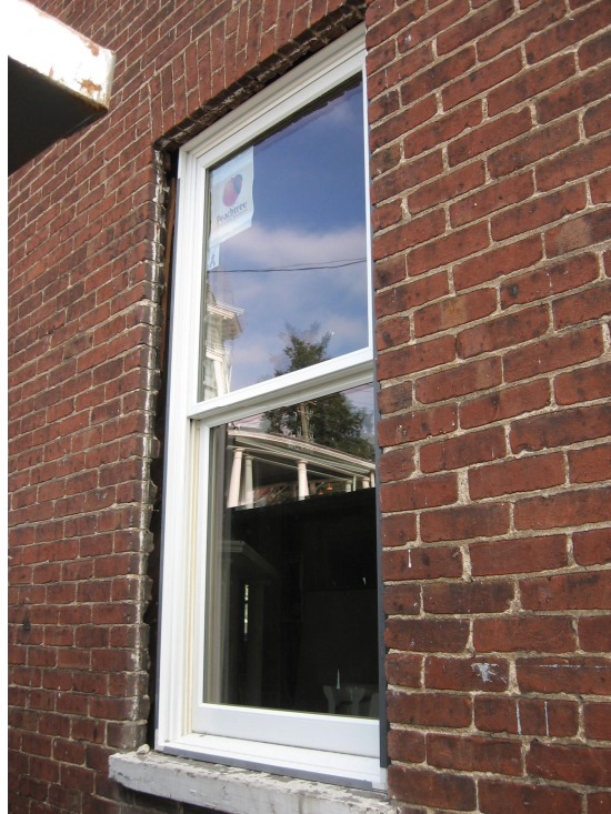
Example of a vinyl clad window approved by the Commission in Roanoke, Virginia
