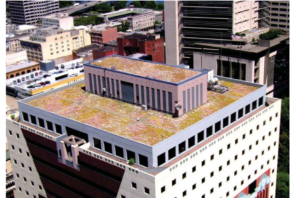
Portland, Oregon has developed numerous incentives for green roofs, green streets, and other green infrastructure which has reduced the cost of city infrastructure.
