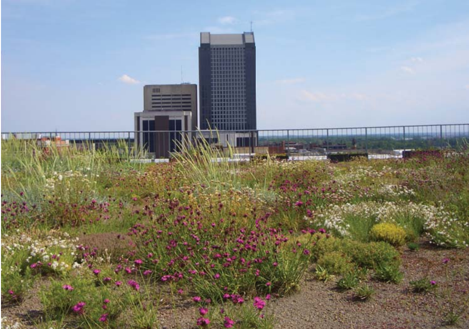
The green roof atop the Lazarus Building retains and slows the flow of stormwater into the City's combined sewer and stormwater system.
