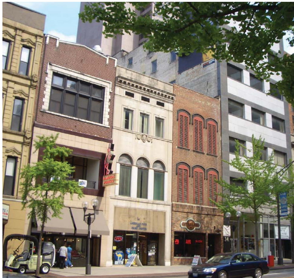
High Street features a mix of modern office towers and older, traditional storefronts.
