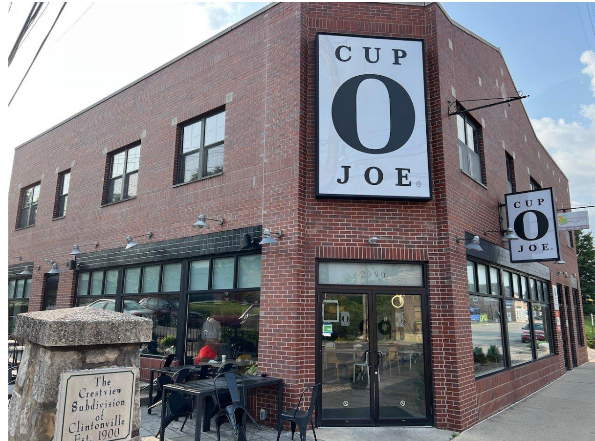
Project built under Urban Commercial Overlay with reduced parking requirements
