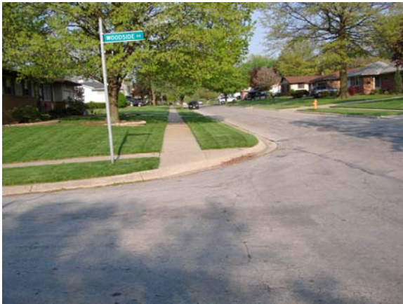
The lack of ADA ramps throughout the neighborhood makes it difficult for senior and disabled residents to navigate the neighborhood.
