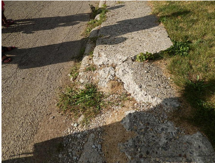
Deteriorating sidewalk.
