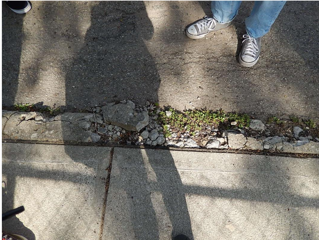
Deteriorating curb.
