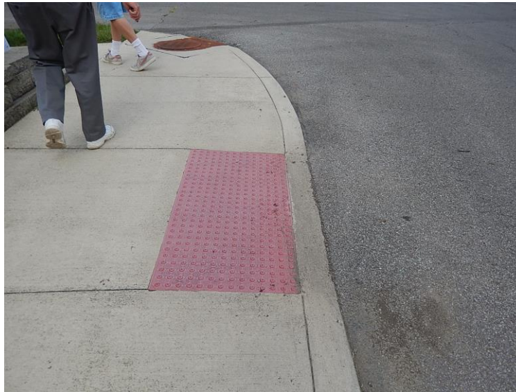
ADA ramp present.
