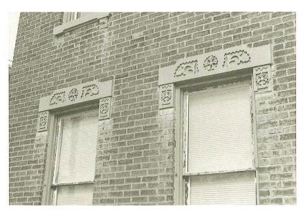
[Photo 33] Although many have been painted over the years, cut-stone lintels such as these were designed to remain unpainted.
