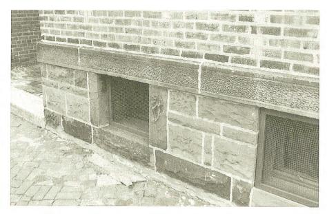
[Photo 2] A rock-faced limestone foundation with a tooled and edged stone water table.
