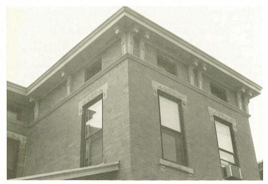
[Photo 3] A traditional Italianate composition of cornice brackets frieze windows, and eave molding.
